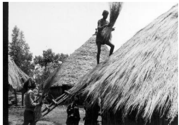
Men repairing the grassed-roof thatch house, Kotekotema village, BPA
