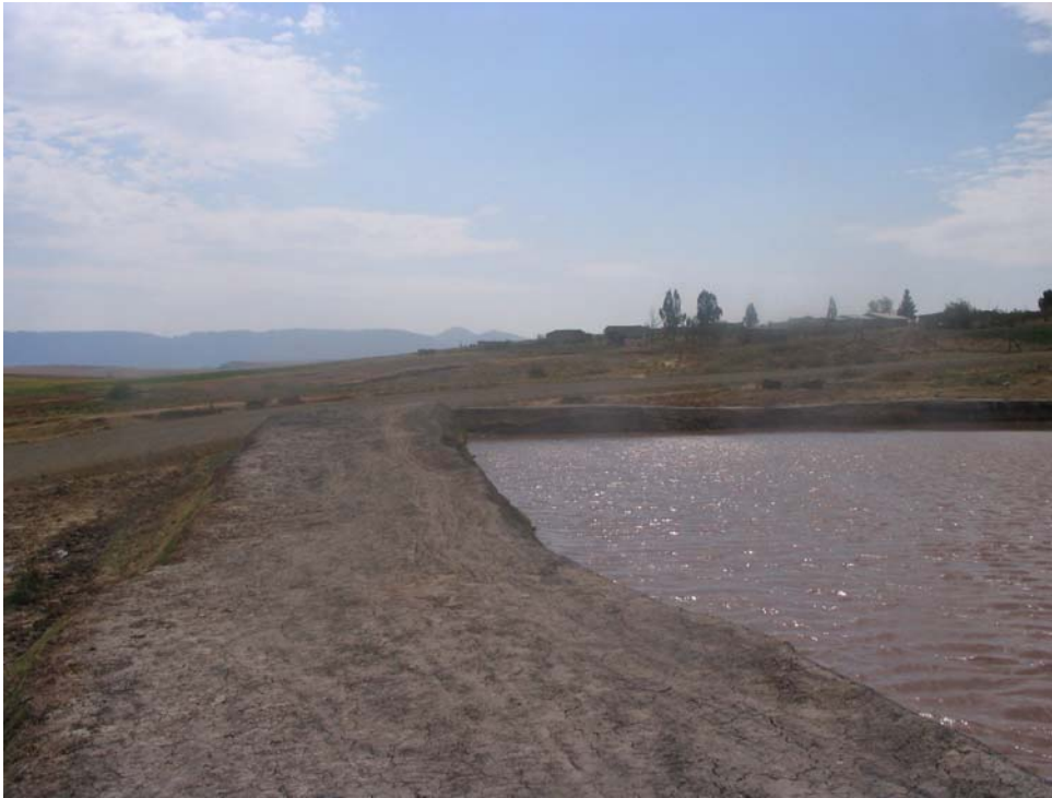
Figure 19: Recently constructed dam
