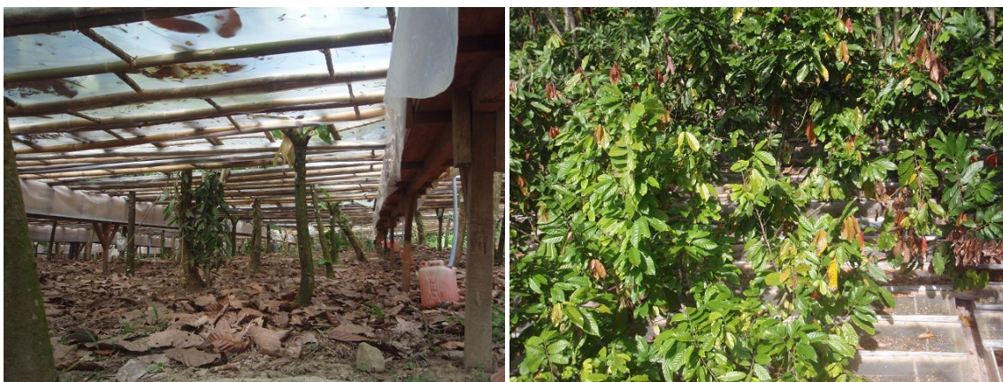
Figure 5: Picture from below and from above the roof installed in the cacao/ Gliricidia agroforest in Indonesia.
