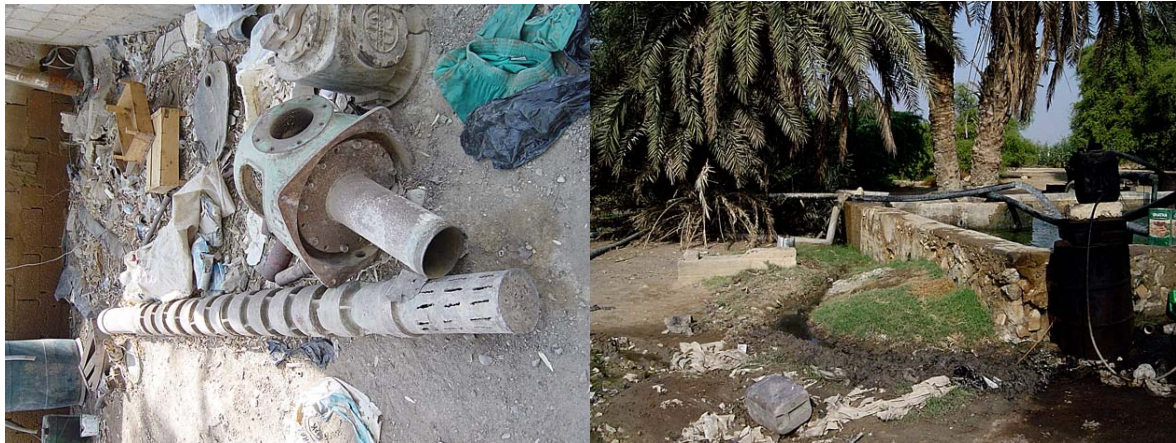
Fig. 4.3-2: Left: torch-cut inflow to the well pump. Right: Irrigation water storage pool.
