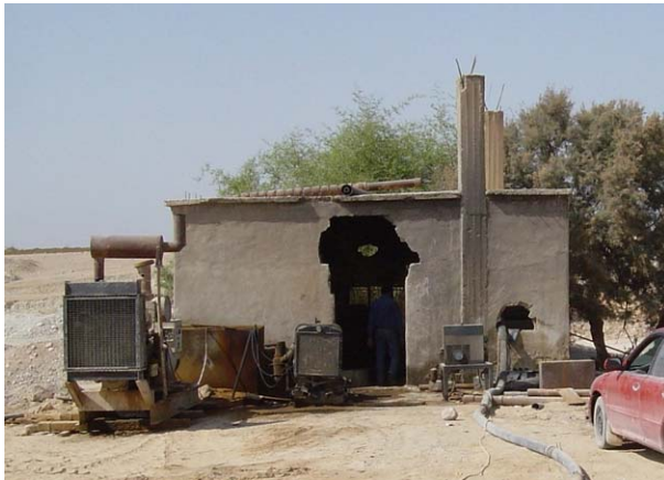
Fig. 4.3-4: Concrete well house. Outside: a former truck engine that is used as a diesel driven generator powering the well pump.
