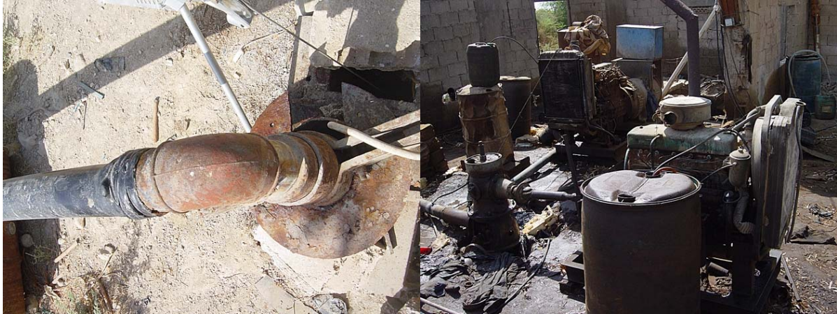
Fig. 4.3-3: Left: Access to the well hole; well pump is held by iron cross bars. Right: Pollution source, deriving from the diesel generators located direct in the vicinity of the open well hole (lower left corner).
