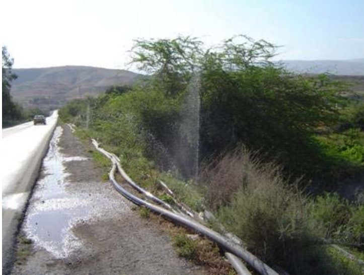
Fig. 3-5: Leaky private off-farm irrigation network near Kafrein.
