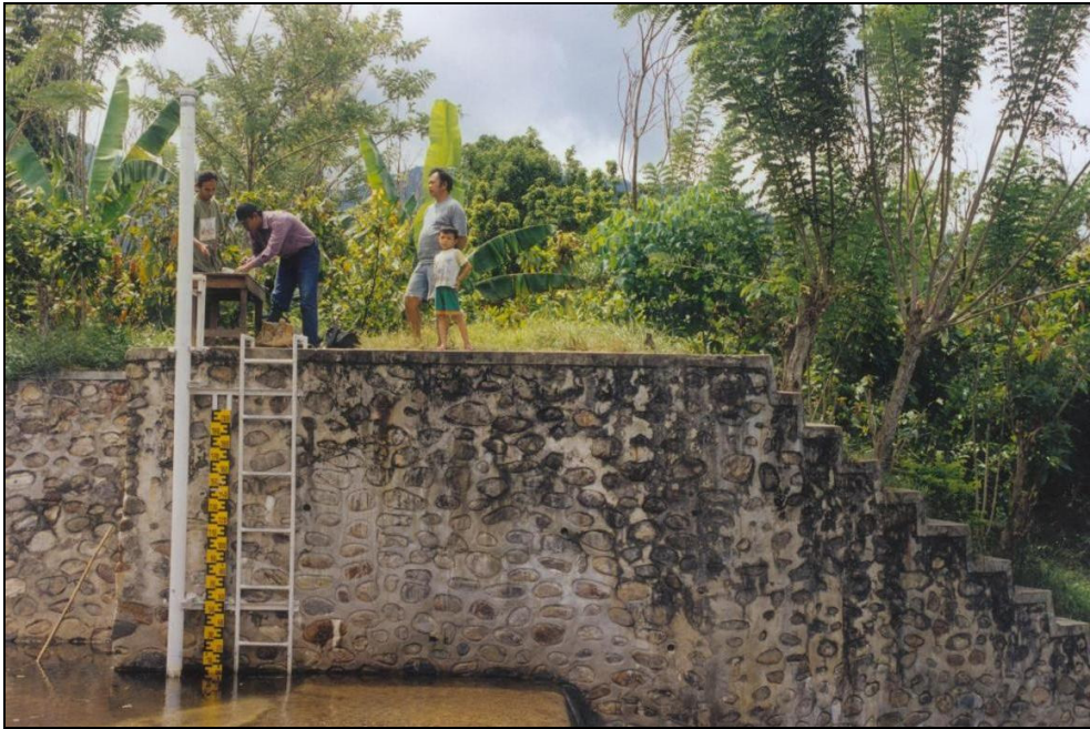
Appendix A. 1: Takkelemo gauging station equipped with a float operated shaft encoder with integral data logger.
