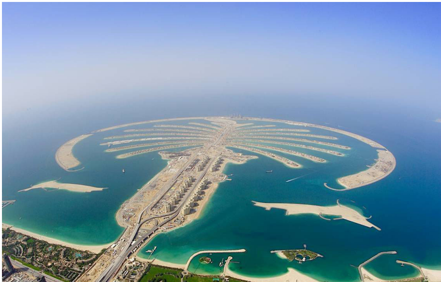
Figure 1: The Palm Jumeirah is constructed in the Persian Gulf in Dubai (copyright Nakheel PJSC ).
