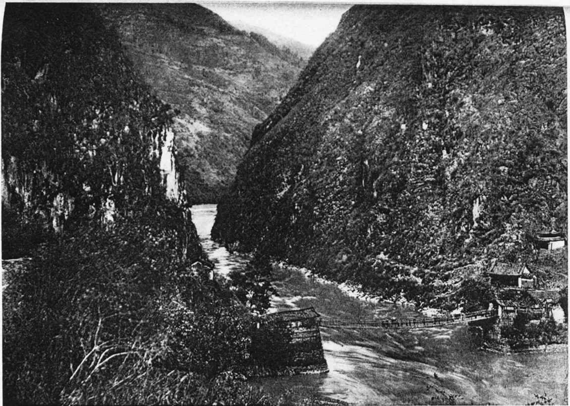
Chain Bridge over the Mekhong between Yung Chang and Tali The bridge sways with mule traffic so that the animals have to be taken over a few at a time. Elephants cannot cross. The caravan track makes a hairpin bend to avoid the precipitous descent.
