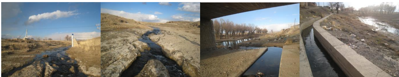
Figure 2-7. The view of Zehtaran River with the hydrometric station. The irrigation channels could change the hydrological characteristics in the basin.
