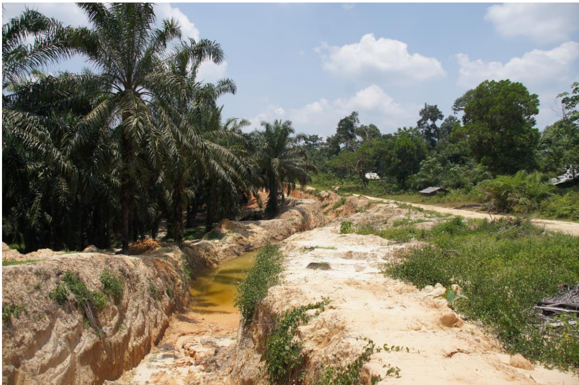
Picture 12 Trench designating the border of the PT Asiatic Persada oil palm plantation
