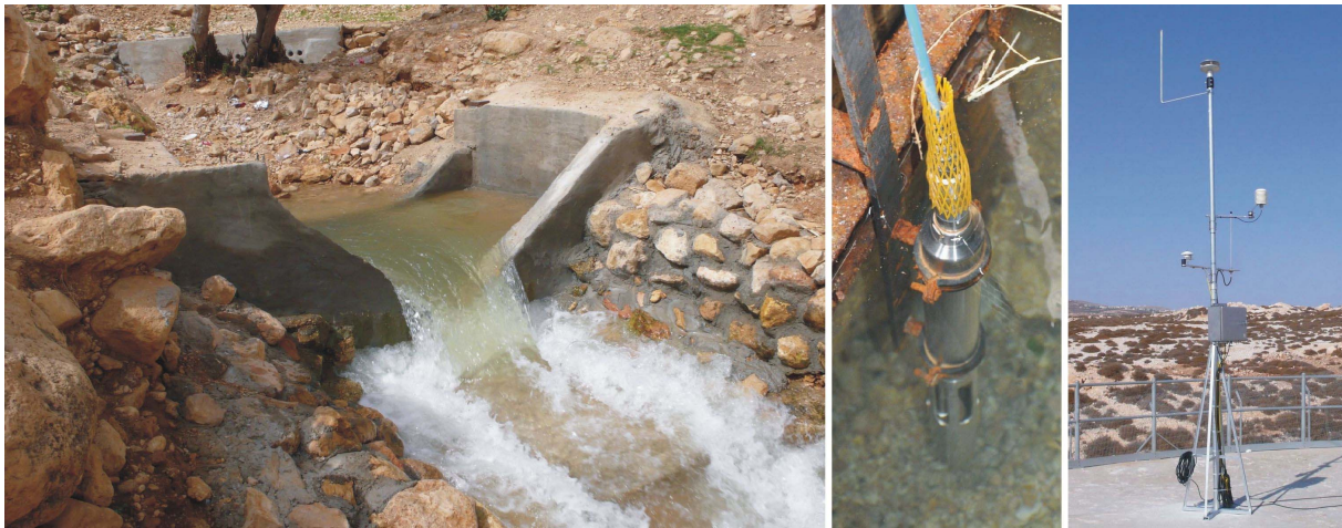
Fig. 2.3: Examples of installations: Left: spring gauging and hydrochemical parameter monitoring station at the Auja spring. The weir was constructed for the research. The spring tapping structure in the background was profoundly rehabilitated. From the structure, an underground pipe leads to the weir. In the structure, the multiparameter-probe is installed (middle). Flow at time of picture was about 500 \text{ l s}^{-1} . Right: Meteorological station on top of a water reservoir.
