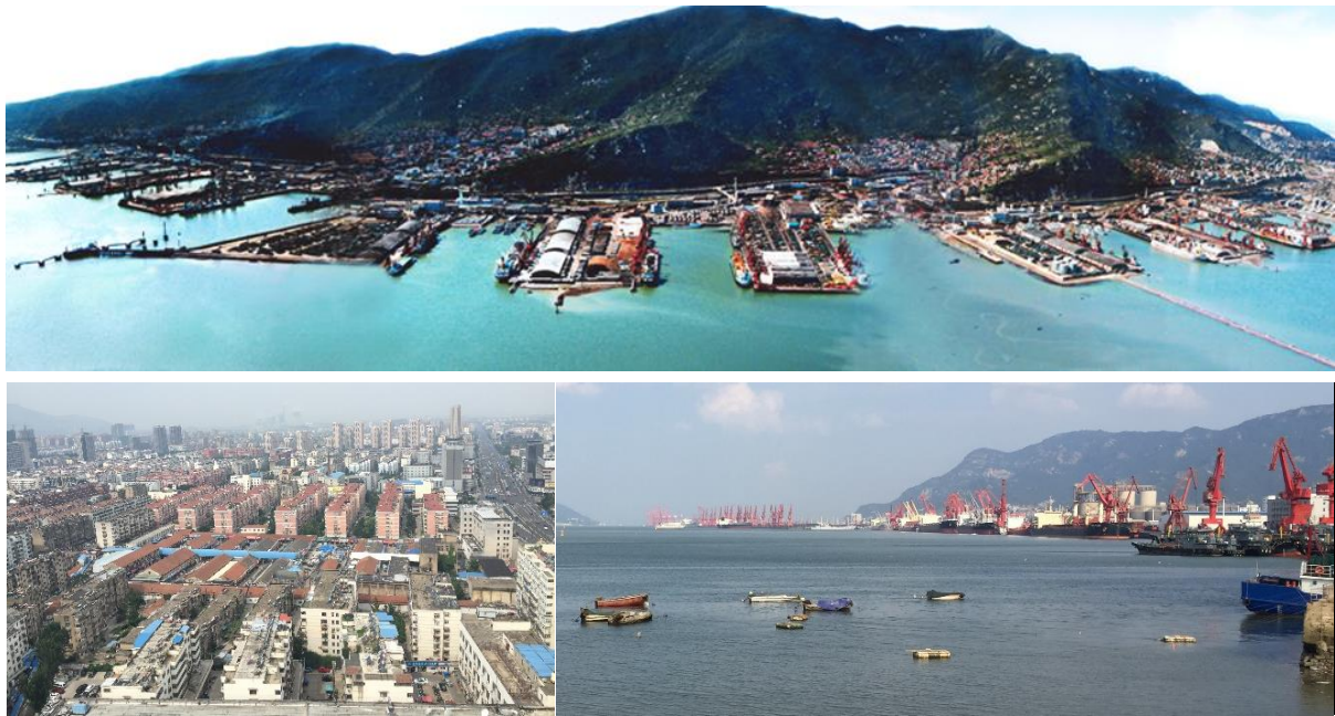
Fig.1.8 Rapid development in Lianyungang
