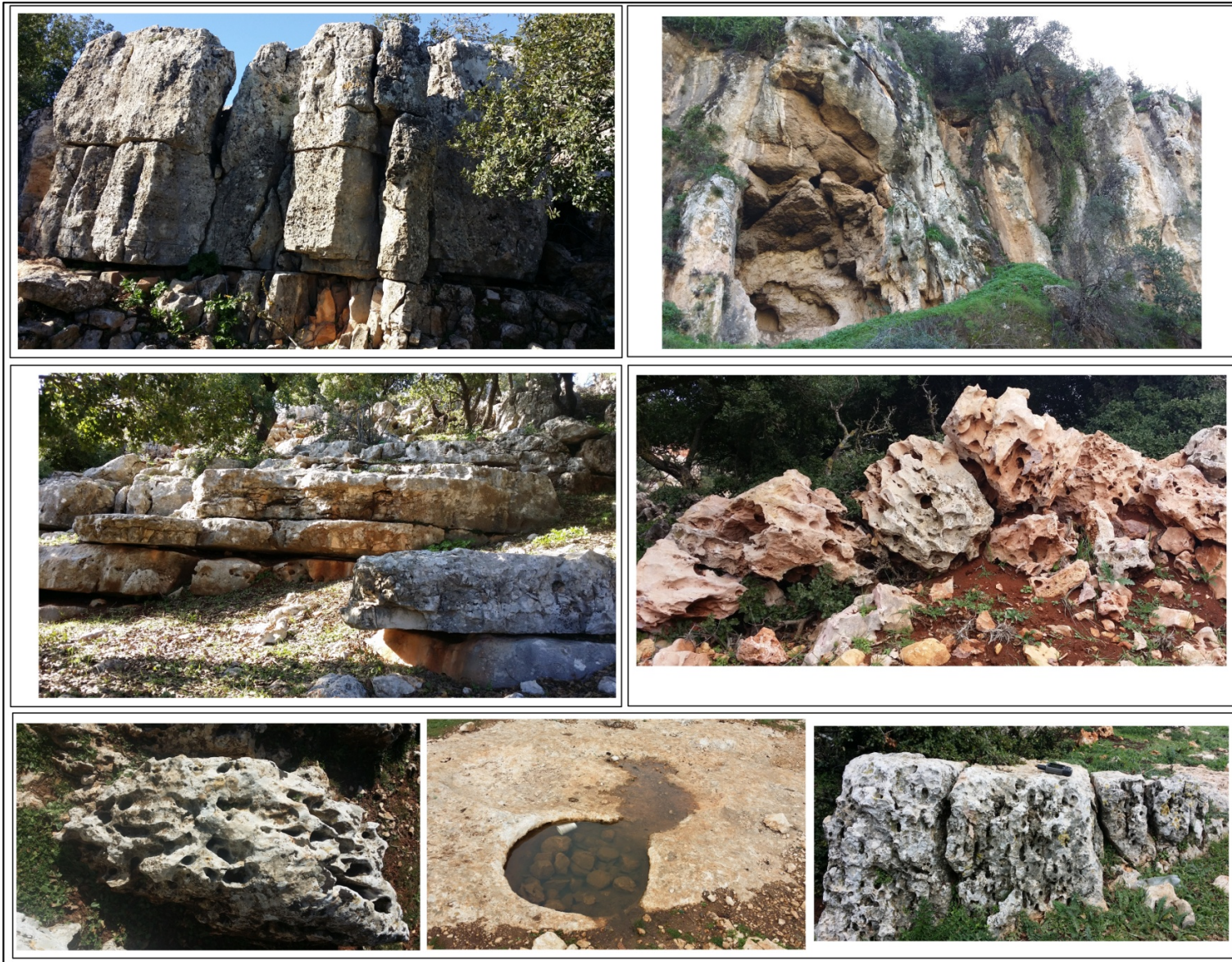
Figure 2-25: Fracturing and dissolution of limestone rock formations (photo source: Ibraheem Hamdan).
