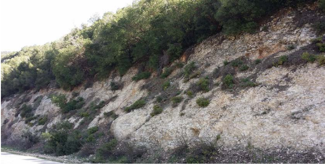
Figure 2-19: Shu'ayb geological formation (A5/6) outcrop in the study area (photo source: Ibraheem Hamdan).
