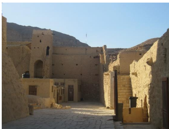
Fig. 1.11: The front of the library building at St Paul's Monastery (to the right). (Photo courtesy of Ayman Na'im).
