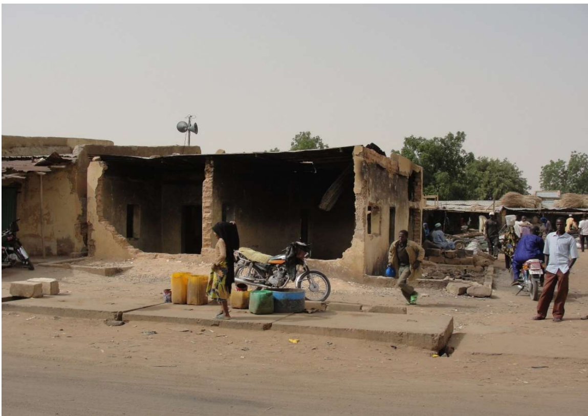
Figure 9: Burned-down police station at the main market. Photo: Jannik Schritt
