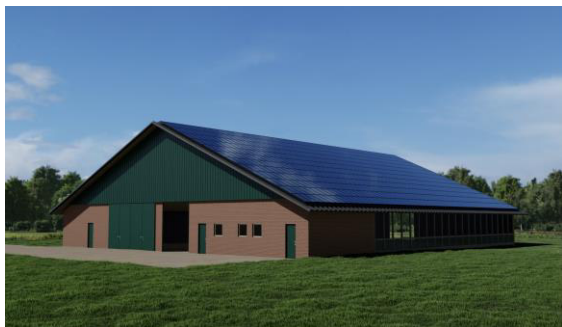
Figure 4. Dairy barn with rooftop solar panels
