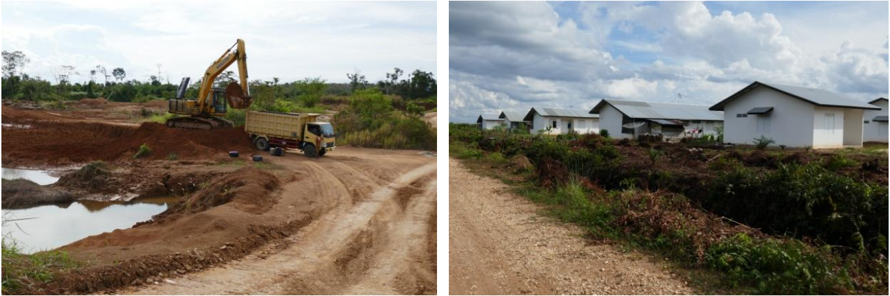
Fig. 2 and Fig. 3: Soil pit (left picture) where mineral soil is being sold to build housing foundations in the peatlands (right picture).
