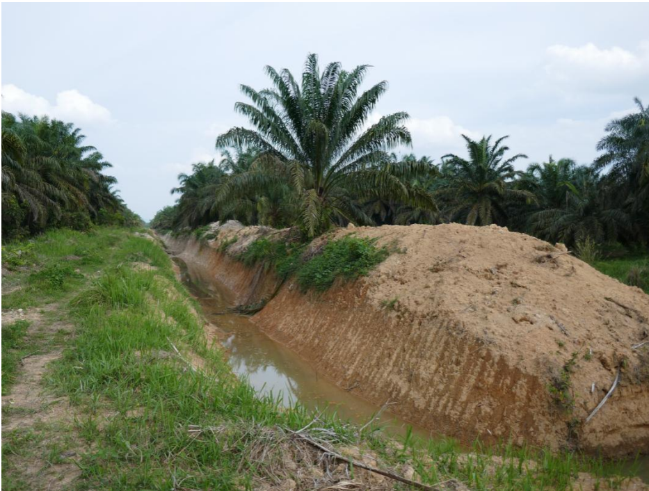
Fig. 2: Recently built flood control dam on an agro-industrial oil palm plantation.:
