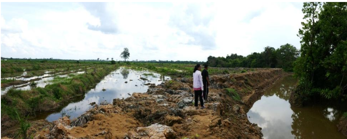
Fig. 6: Recently built flood control dam in the Air Hitam sub-district.
