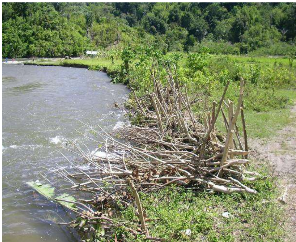
Figure 5.8: Protective water barrier.
