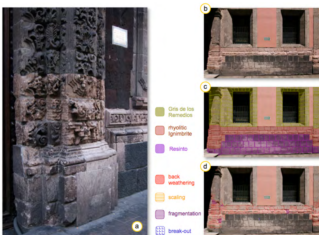
Figure 48: a) Weathered and replaced building stones at the ground level, b) mapping area, c) lithographic mapping, and d) map of damages.
