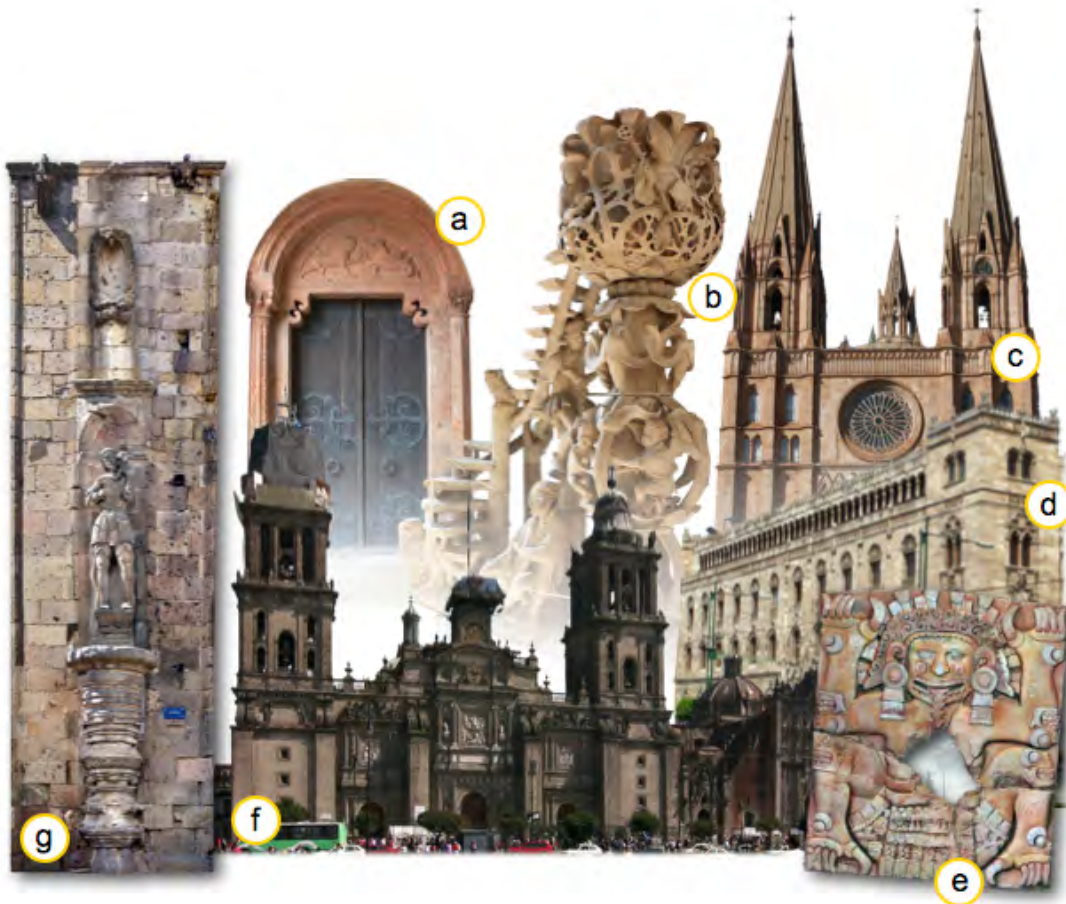
Figure 2: Volcanites used as building stones and for artwork: a) Rochlitz Tuff, RP (portal at monastery Wechselburg/ Germany), b) Hilbersdorf Tuff, HD (tulip pulpit in cathedral of Freiberg/Germany), c) Cantera Rosa San Miguel el Alto, CR (cathedral Arandas/Mexico), d) Blanca de Pachuca Tuff, BP (Palacio Postal Mexico City), e) Tenayocátetl Tuff, TY (Aztec sculpture Tlatecuhtli, Templo Mayor, Mexico City), f) Chiluca, CH, and Cantera Gris de los Remedios, GR (cathedral of Mexico City), and g) Cantera Amarilla Tuff, CA (Santa Monica Church, Guadalajara/Mexico).
