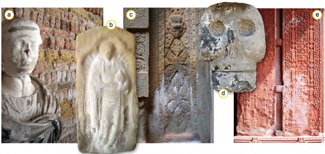
Figure 153: Salt weathering is a main weathering form that occurs on historical monuments worldwide and the contamination can have various sources. a) Weathering of marble and brickstone due to marine salt contamination in Venice/Italy, b) a salt contaminated tomb plate due to magnesium sulphate salts created by the binding material of the sandstone and industrial pollution, c) salt weathering at a temple of Angkor/Cambodia due to bat guano, d) salt weathering of a skull at the Templo Mayor in Mexico City due to salt contamination within the groundwater and rising dampness and e) salt weathering due to contamination by pigeons at the Fatipur Sikri Temple/India.
