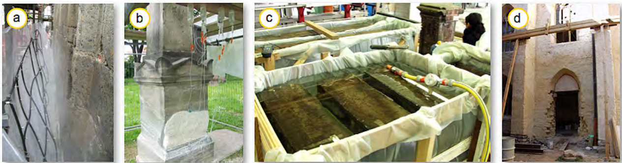
Figure 34: Different methods of desalination. a) sprinkling, b) combined injection and poultice method, c) desalination bath and d) poultice.
