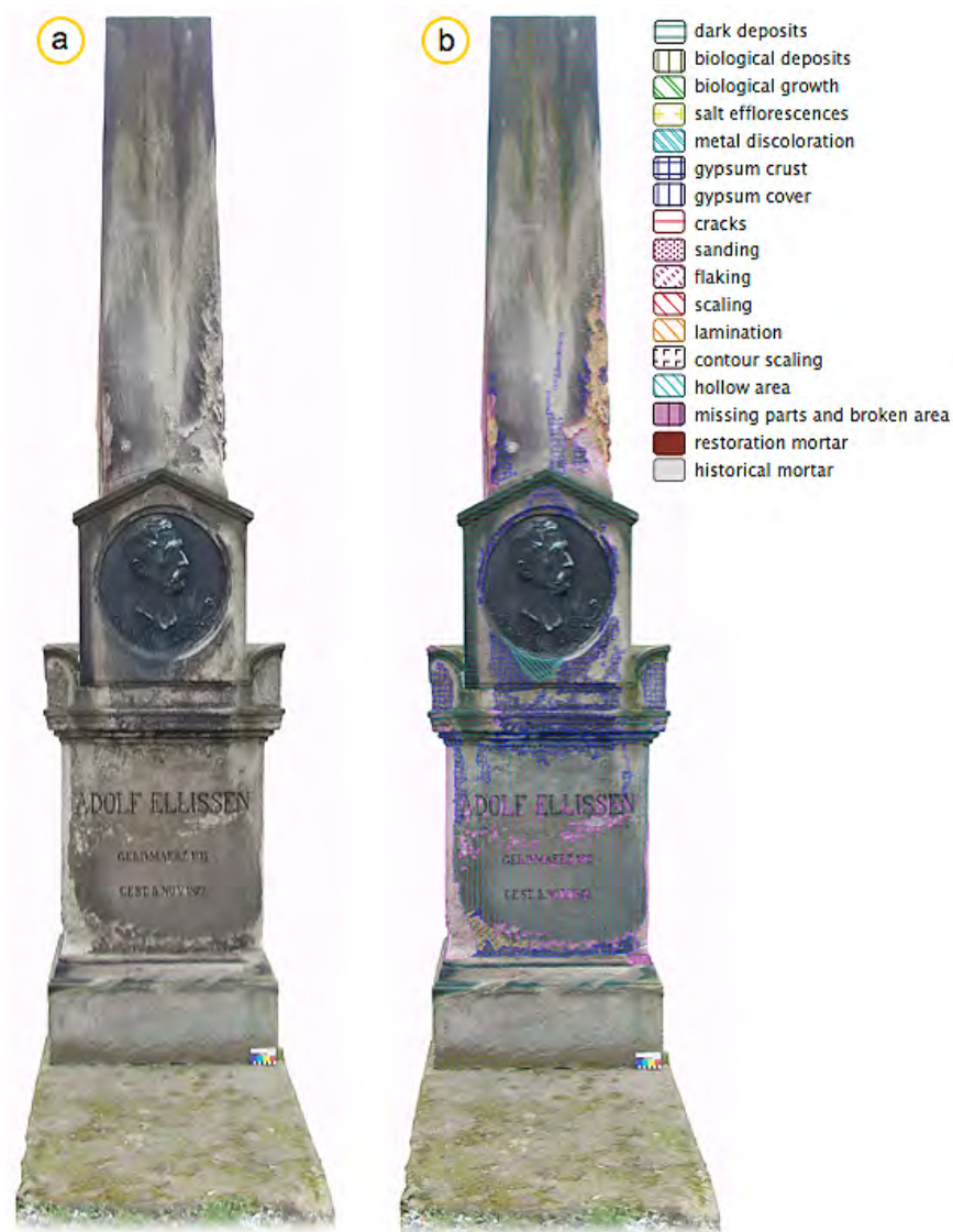
Figure 95: The Ellissen-Tomb. a) The tomb before conservation/restoration. b) Damage mapping of the tomb.
