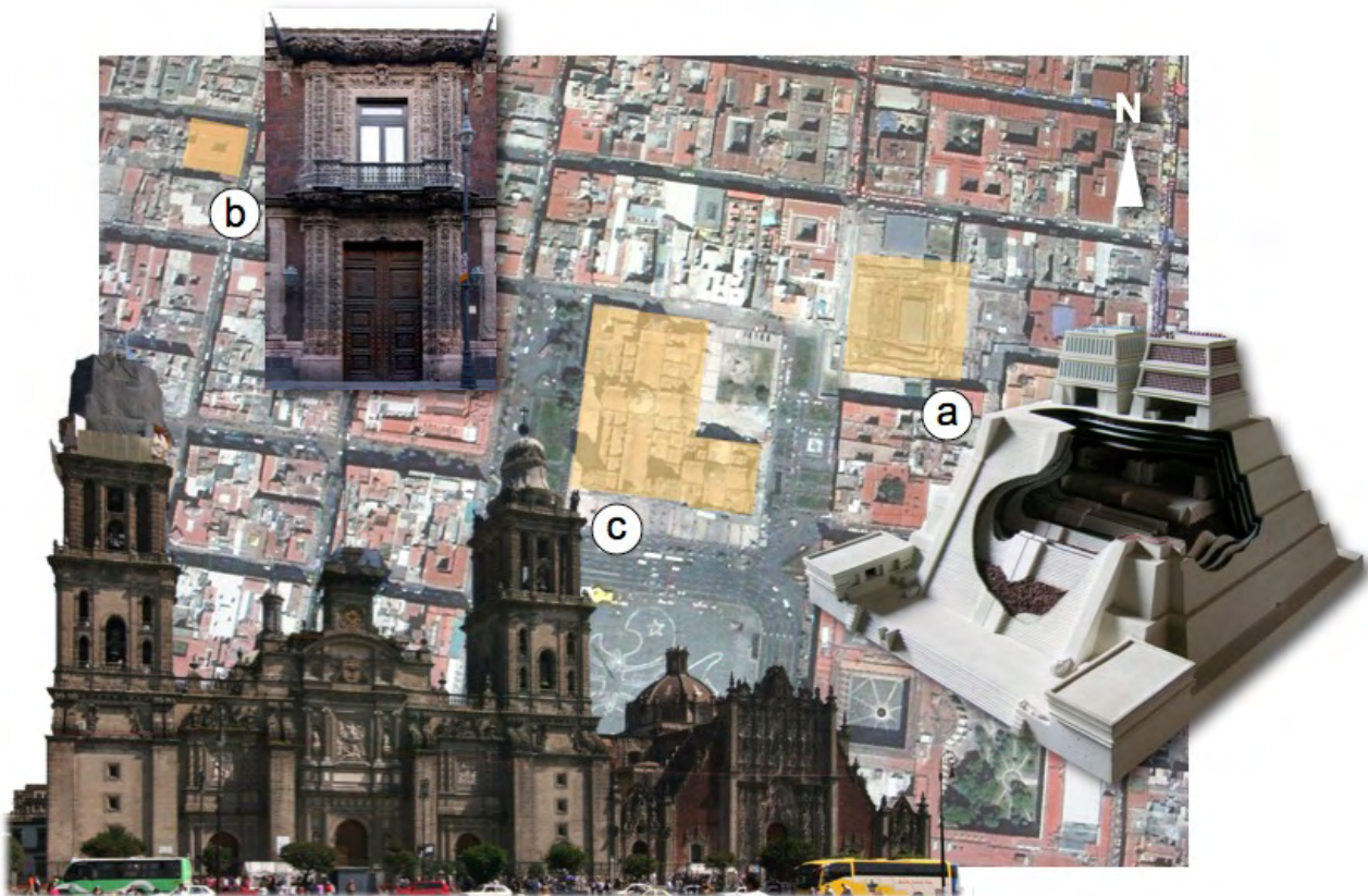
Figure 42: The investigated buildings within the historical center: a) location and model of the Templo Mayor, b) the palace of the dukes of Heras Soto and c) the Metropolitan Cathedral with the left tower under restoration.
