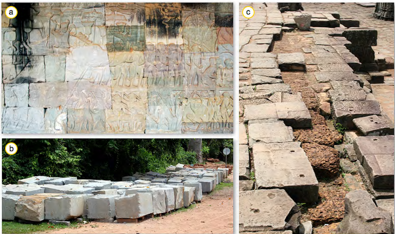
Figure 123: a) Different colored Angkor sandstones at the Bayon Temple. b) Fresh quarry material for the restoration of the Phnom Bakheng Temple. c) Laterite masonry underneath the sandstone plates of the Phnom Bakheng Temple.
