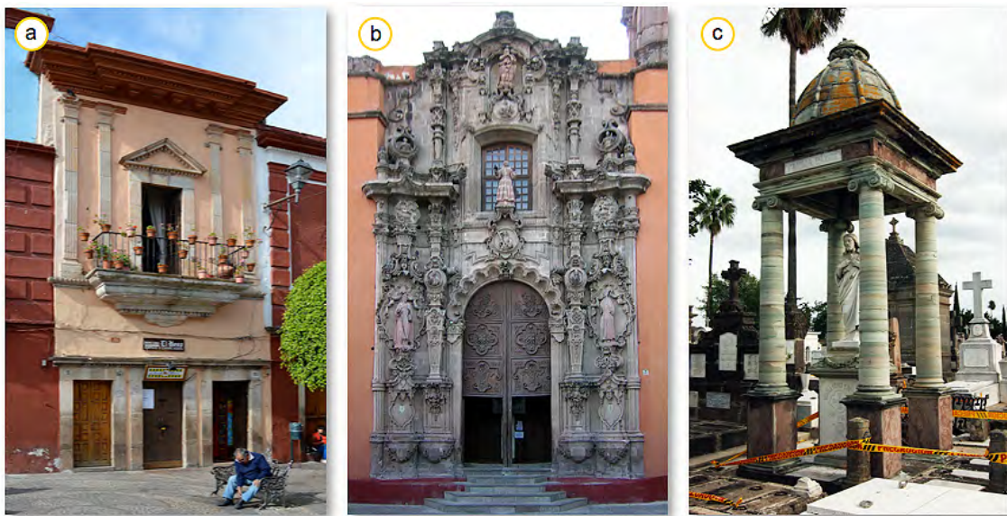
Figure 58: a) A 19 th century house in the historical city of Guanajuato with decorative parts made from Loseros Tuff. b) The portal of the San Diego Church in Guanajuato mainly made from Bufa Tuff c) Monumental tomb at the Mazquitlan Cemetery in Guadalajara made from Loseros Tuff.
