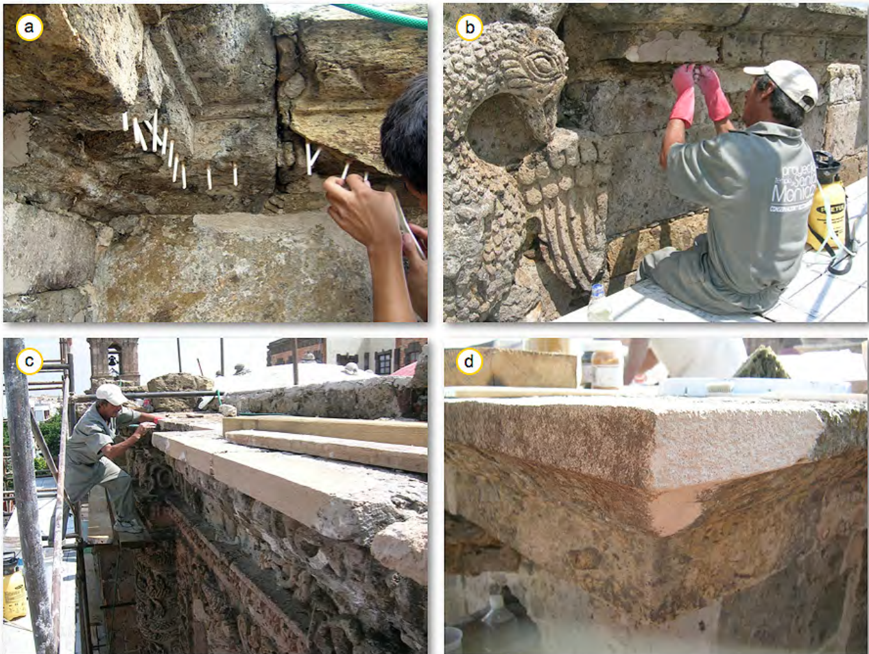
Figure 183: a) Glueing of fiberglass sticks within areas of missing parts of the tub profile. B) Fillings with lime mortar, and c) re-profiling. d) Fresco-like retouch of the restored areas.
