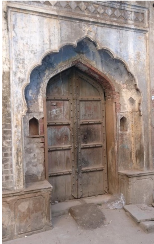
Figure 4.6: A locked dilapidated Muslim house. Source: Author.
